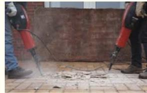
Chainsaws, jackhammers as well as other tools and heavy equipment create noise levels that can damage workers' hearing—especially after prolonged exposure. Pre-molded or formable ear plugs are usually the best choice but acoustic foam-lined ear muffs that tightly seal against the head can work well too.
