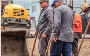
Workers should protect their full legs, full arms, and torso against cuts, scrapes, burns and other superficial injuries with thick, flexible work pants and shirts. These should fit closely and never be baggy while allowing for maximum mobility.
