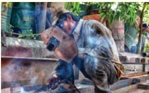
Safety glasses or face shields should be worn whenever there is a risk of flying debris or harmful dust getting in the eyes. Cutting, grinding, welding, chipping and nailing are some activities that necessitate protective eyewear. Along with basic safety glasses, some other protective wear for the face include welding shields, chemical splash goggles, and dust goggles.
